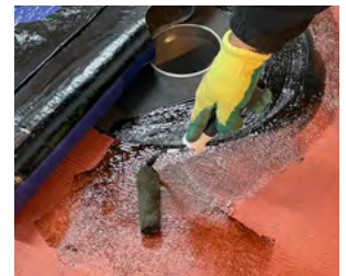
2. Apply primer to the upper surface of the membrane flange and underlay
