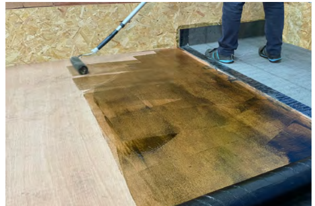
2. The prepared substrate is primed using Icopal SA Primer
