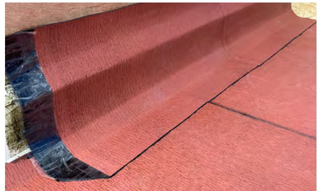
4. TorchSafe TA Detailing Underlay installed to upstand
