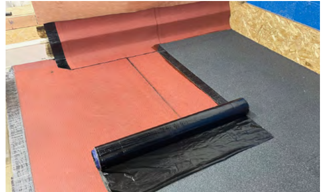
1. Set the rolls of TorchSafe TA Mineral Capsheet
