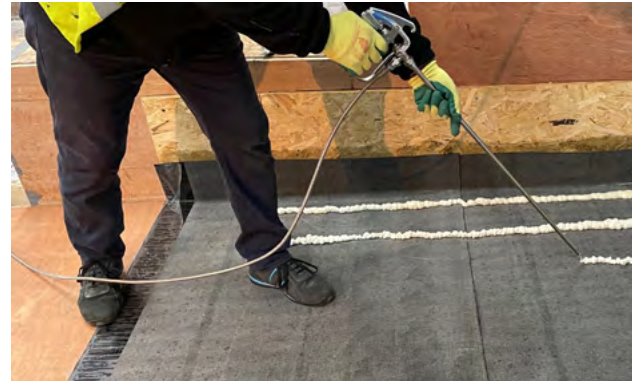
1. Apply minimum 30mm beads of Icopal Insulation Spray Adhesive
