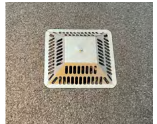
4. Weld the capsheet to the circumference of the outlet aperture and install the leaf grate
