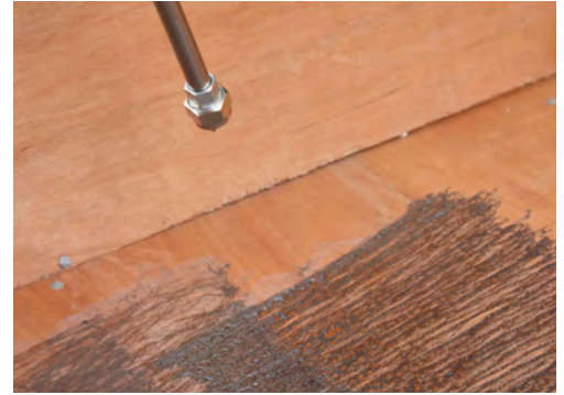
Spray "Cobweb" application of primer
