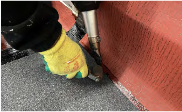
1. Hot air weld the field area capsheet to the detailing underlay
