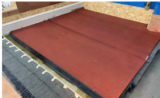
3. Pyrobar Underlay to field area
