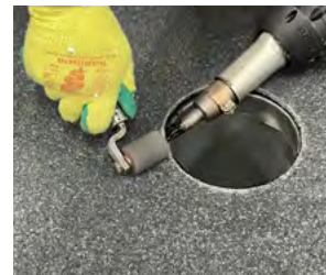
4. Weld the capsheet to the circumference of the outlet aperture and install the leaf grate
