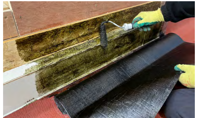
2. Apply primer to upstand detail
