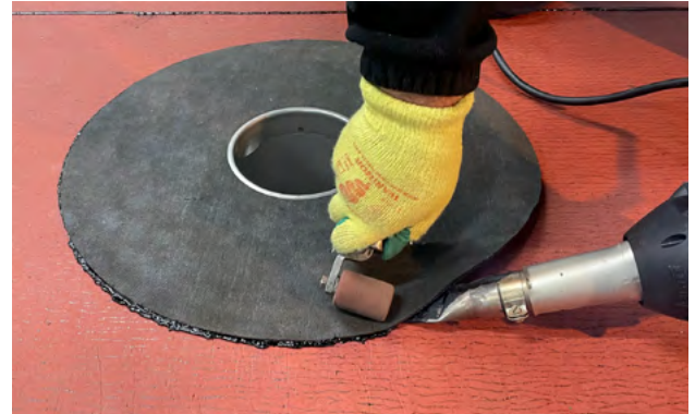
1. Weld the membrane flange to the Pyrobar Underlay
