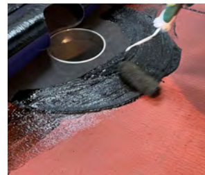
2. Apply primer to the upper surface of the membrane flange and underlay
