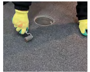
3. Lay the TorchSafe TA Mineral Capsheet above the primed membranes
