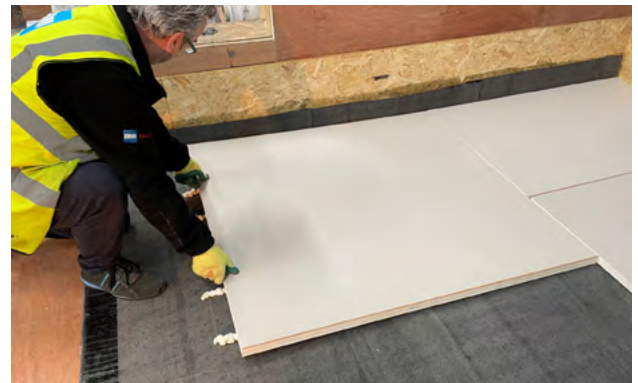
2. Lay the insulation board into the adhesive
