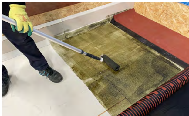
1. Apply primer to the upper surface of the installed insulation
