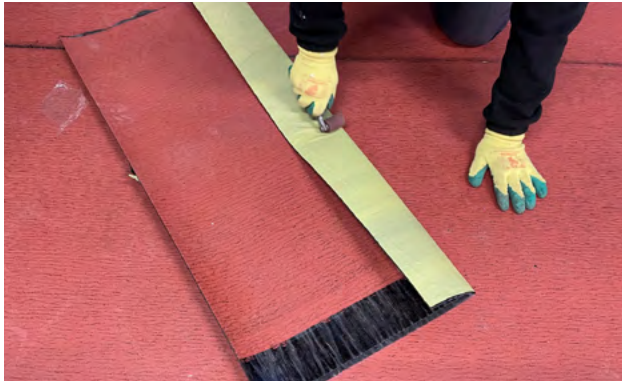
1. Cut and pre-crease detailing underlay
