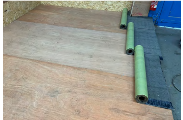
1. Rolls of Vapour Control Layer are set in position prior to substrate priming
