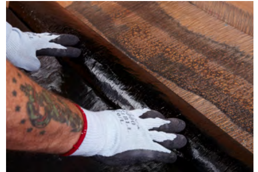
Apply membrane with downward pressure
